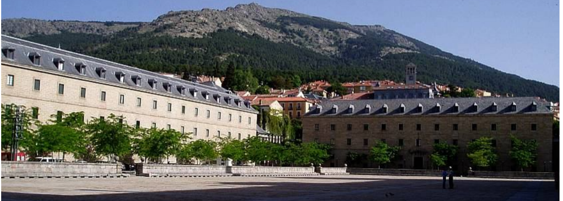
Exterior and interior Courtyard
